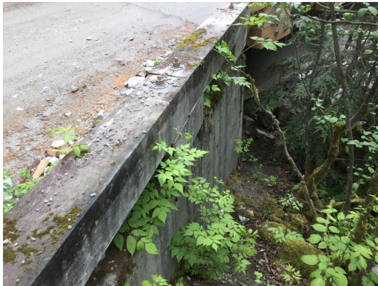
Wingwall downstream right bank
