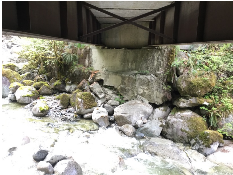
Left Bank Abutment when facing downstream
