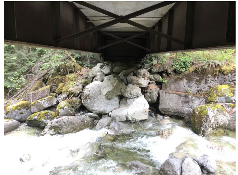
Right Bank Abutment when facing downstream
