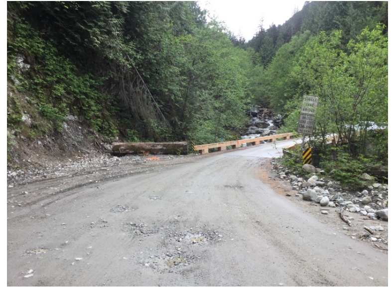
Approach from Right Bank when facing downstream
